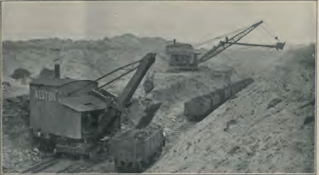
FIG. 3—In the distance is a machine for digging the cover and discharging it direct to the dump; in the foreground the machine is digging iron ore and discharging it into wagons.
